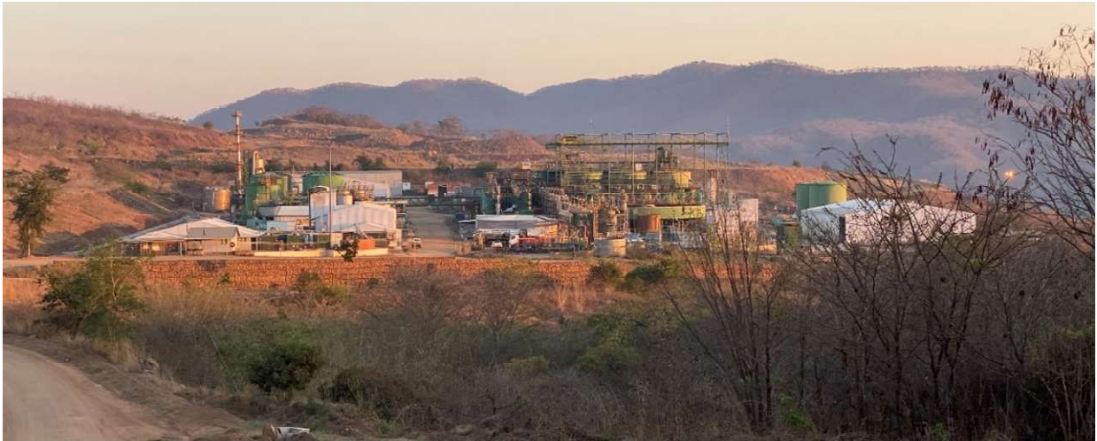
Figure 2: Kayelekera Process Plant and Surrounds – October 2019
